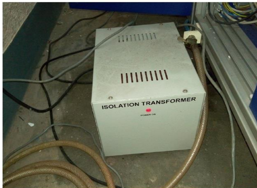
Fig. 3.2. Photographic view of isolation transformer
