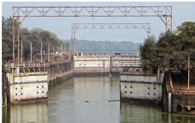
Fig. 9.1: Existing Navigation lock gate at Farakka (source- http://www.srlinson.blogspot.com )
