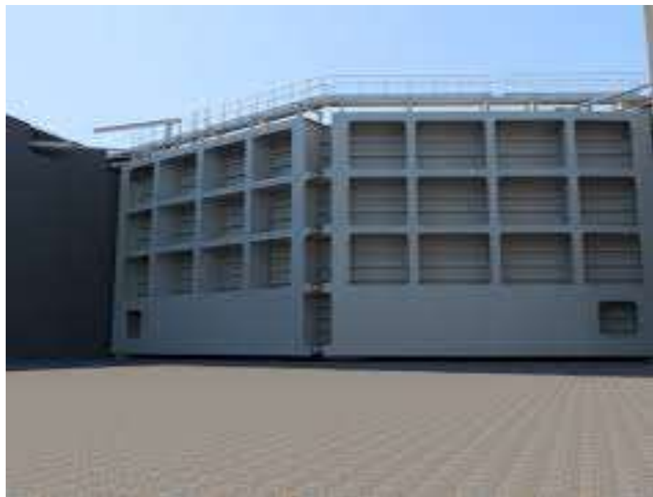
Fig. 8.4: Front view of mitre gate (source- http://www.sbe.be/en/reference/navigational-lock-farakka )
