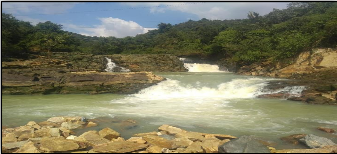
Photograph 3.1: Tail race channel of Maithon Hydel Power Station
