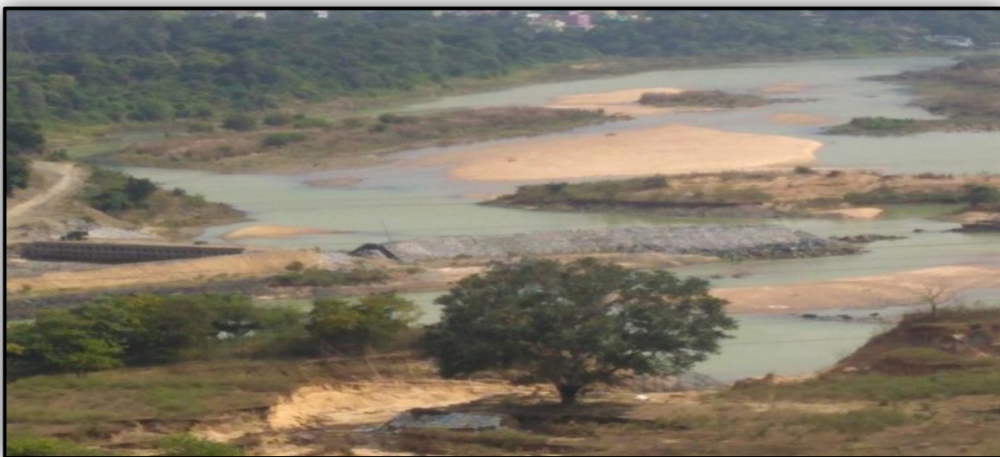
Photograph 3.2: Discharge out let of the Maithon Hydel Power Station
