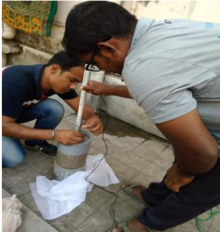
Fig. 66: covering new cloth filter on perforated pipe
