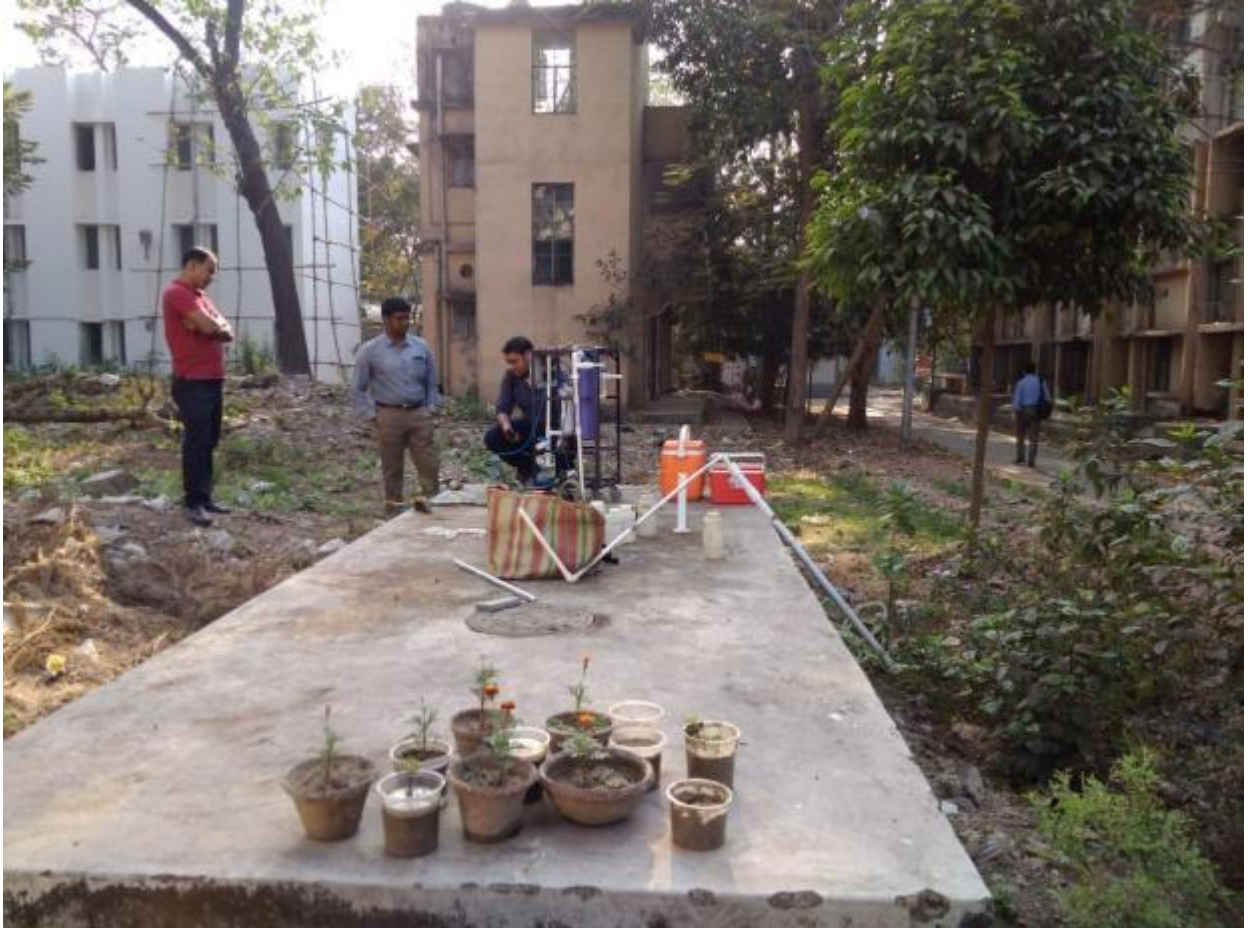
Fig. 4: Septic Tank at Site 3.
