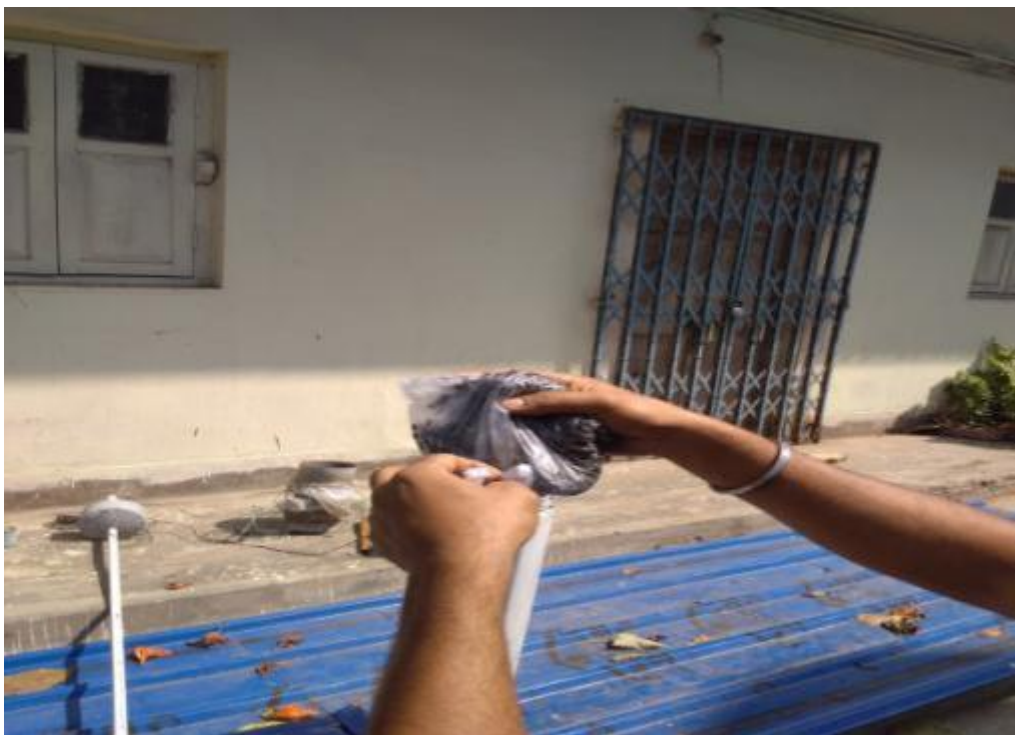
Fig. 63: Installing new GAC
