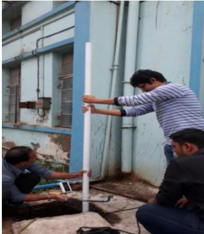
Fig. 29:- installation of perforated pipe
