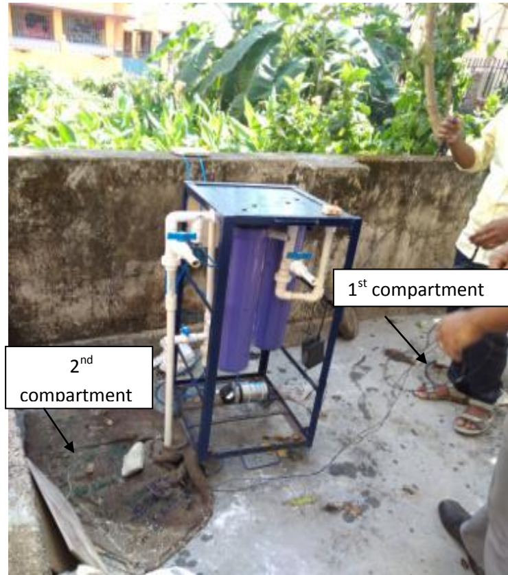
Fig. 68: Installing machine at Survey park
