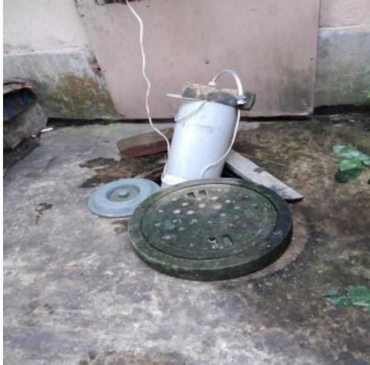
Fig. 15: Brick is placed upon the pipe to resist its upward movement
