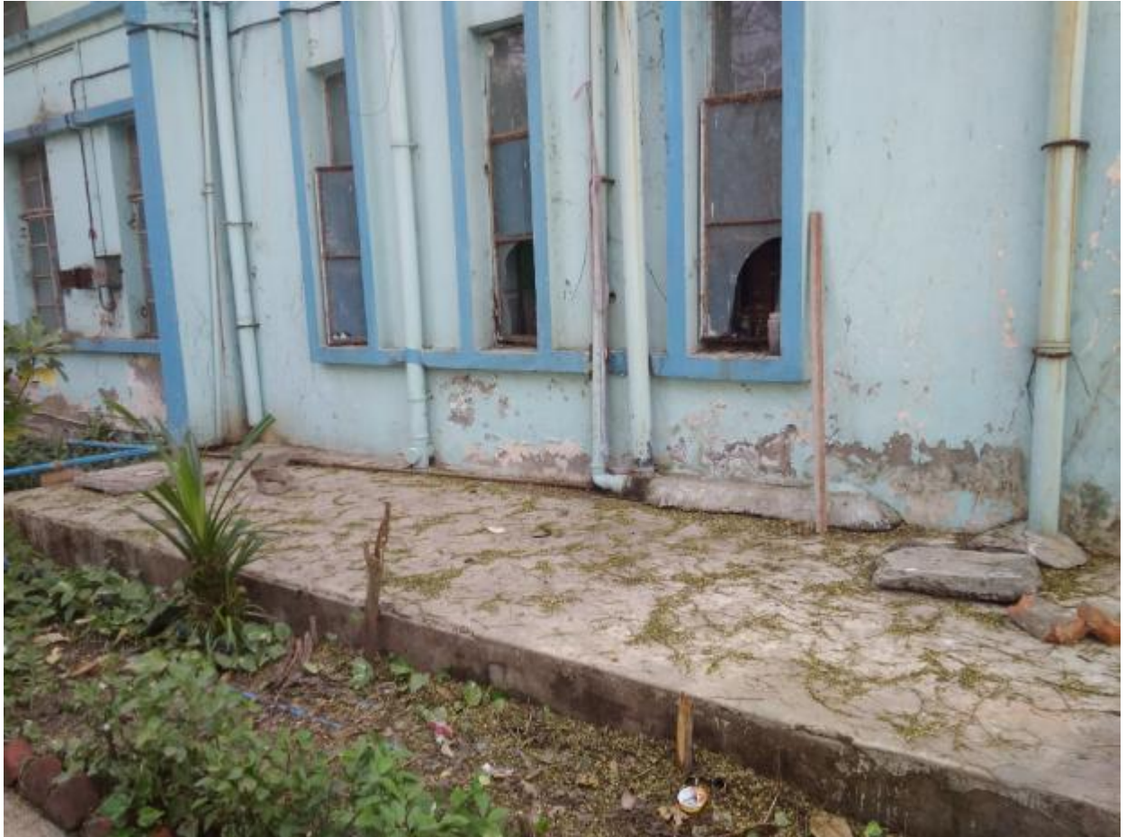
Fig. 3: Septic tank at Site 2.
