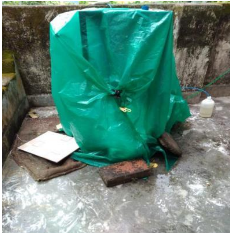
Fig. 69: Machine was covered due to heavy rain
