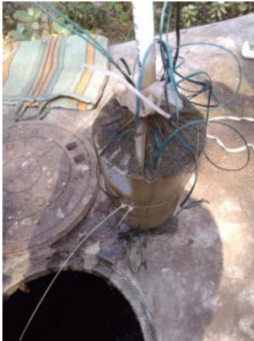
Fig. 48: Perforated pipe after 3days of operation
