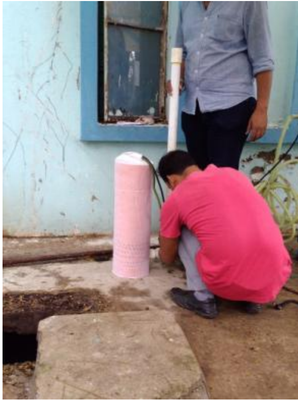
Fig. 38: Perforated pipe covered with cloth filter
