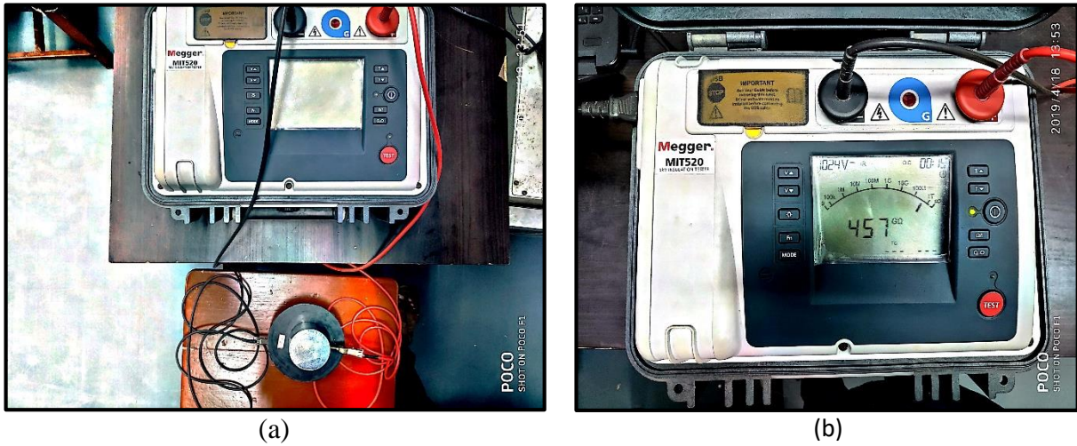
Fig. 5.2. (a) Setup to Insulation Resistance Test and (b) MEGGER MIT520.
