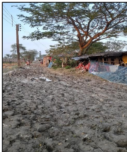
Photograph.2: Condition of the inland road in Mritunjaynagar, Sagar
