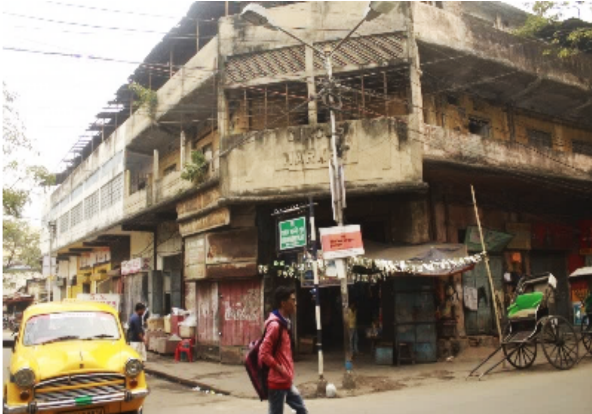
Figure 4-20 : Exterior view of Park Circus market. (Source: Author)
