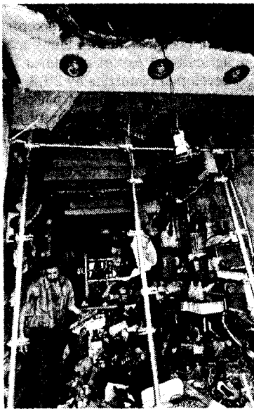
DESTRUCTION: An Iraqi inspects his shop following a roadside blast in central Baghdad on Sunday night.
