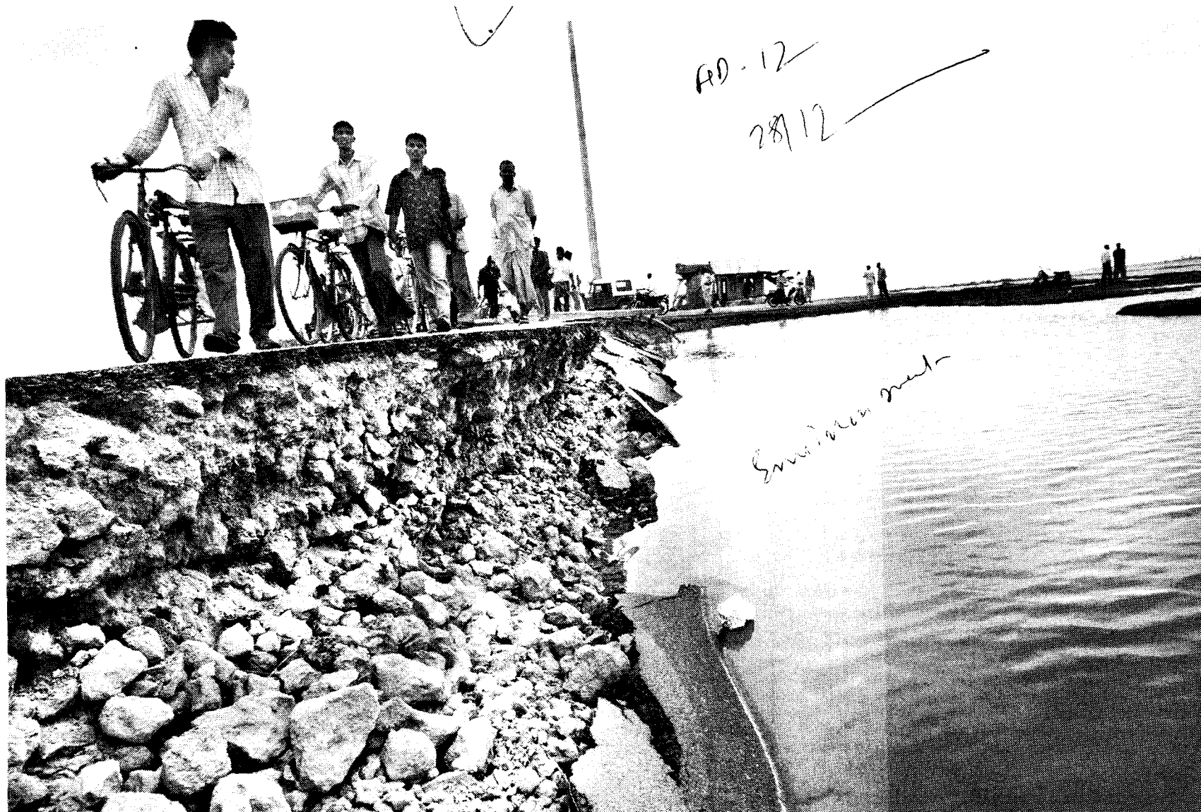
People walk on a road damaged by tsunami waves at Silver Beach area of Cuddalore on Monday. — AP
