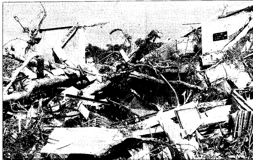
Destroyed living quarters at the Car Nicobar air base, which was washed away on Sunday.
