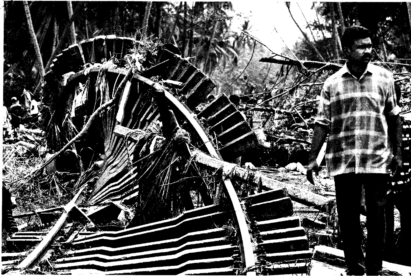
The railway track that was damaged when tidal waves came crashing in Sinigame on the southwestern coast of Sri Lanka on Sunday. A train was washed away leaving 1,000 passengers dead or missing. — AFP
