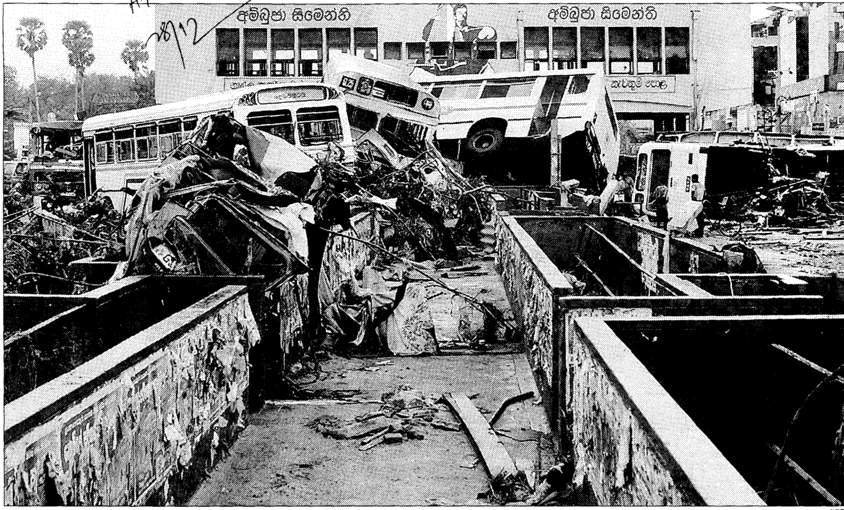
RAZED TO THE GROUND A general view of the destroyed central bus terminal in Galle, 125 km south of Colombo, on Monday.
