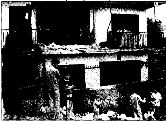
A government office building, on the outskirts of Kathmandu, destroyed in an explosion triggered by the Maoists on Tuesday. — AFP
