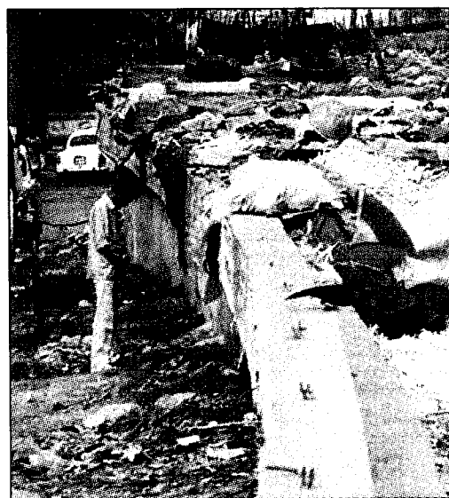
The Kidderpore flyover. Picture by Amit Data
