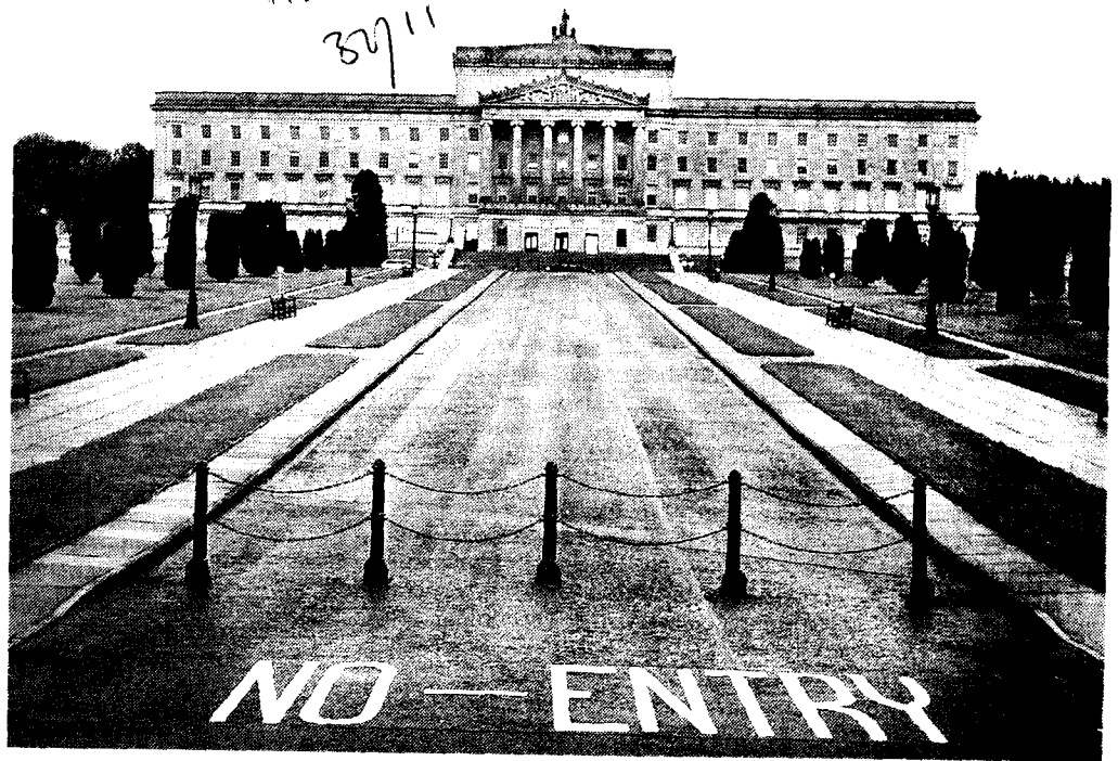
UNCERTAIN FUTURE: The Stormont Parliament Buildings, home of the disbanded Northern Ireland Assembly, in Belfast. — Reuters
