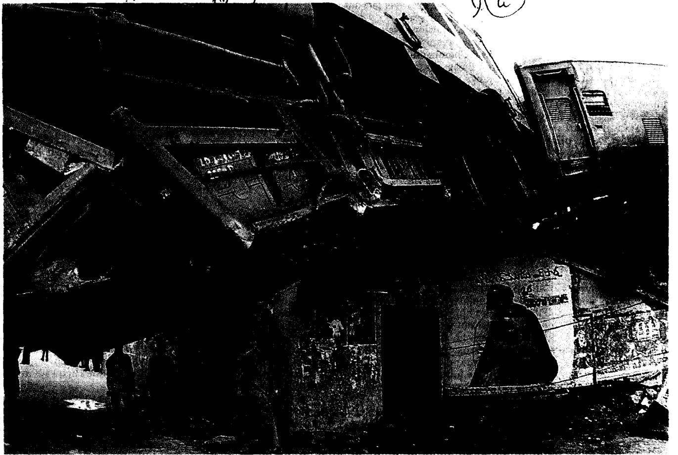
The engine of the Golconda Express hanging precariously after falling off a road underbridge near the Warangal railway station on Wednesday. — Photo: P.V. Sivakumar
