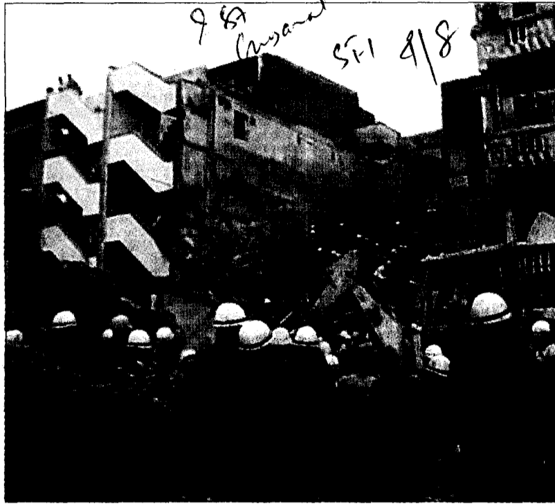
Firemen inspect the debris after the early morning blast. — AFP
