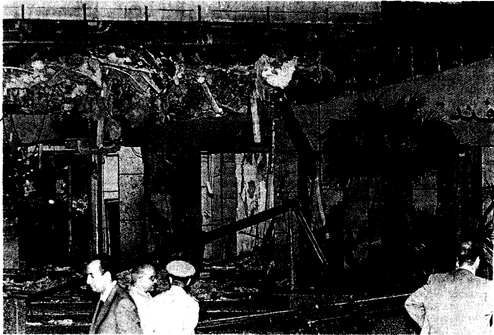
The exterior of a hotel damaged in a suicide bomb attack in Casablanca, Morocco, on Friday. — Reuters
