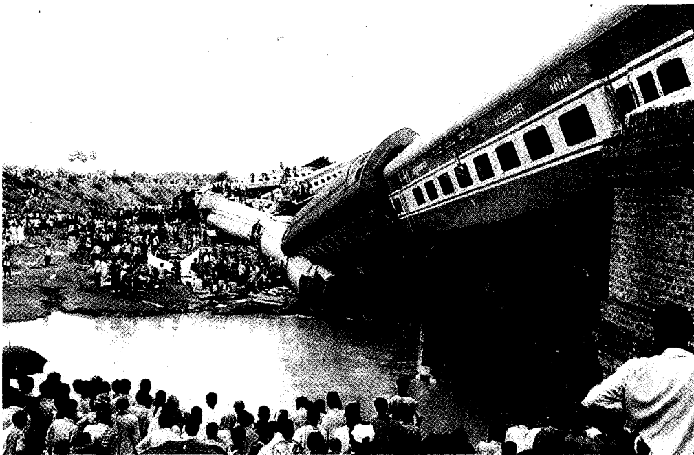
The derailed bogies of the Rajdhani Express at the Dhava bridge near Rafigang, Aurangabad, on Tuesday. — Photo: Ranjeet Kumar (Reports on Page 12)
