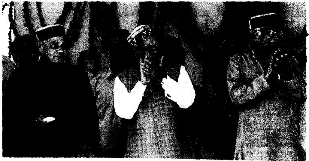
The Prime Minister, Atal Behari Vajpayee, laying the foundation of the Rohtang Pass tunnel at Bahang near Manali on Sunday. The Defence Minister, George Fernandes, (extreme right) and the Himachal Pradesh Chief Minister, P.K. Dhumal, (centre) look on. — PTI
