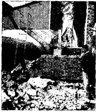
The damaged Coke plant near Kathmandu.
