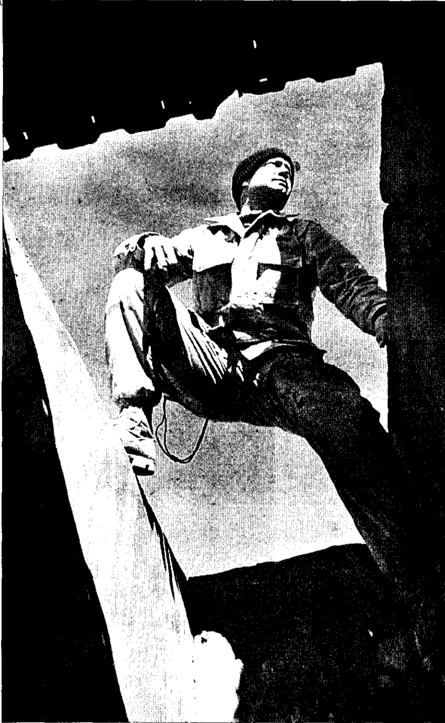
US Navy Seabee Lt Commander Len Cooke climbs upon the roof of a bathhouse next to the Kandahar International Airport to help make repairs to a water system on Thursday. — AP/PTI
