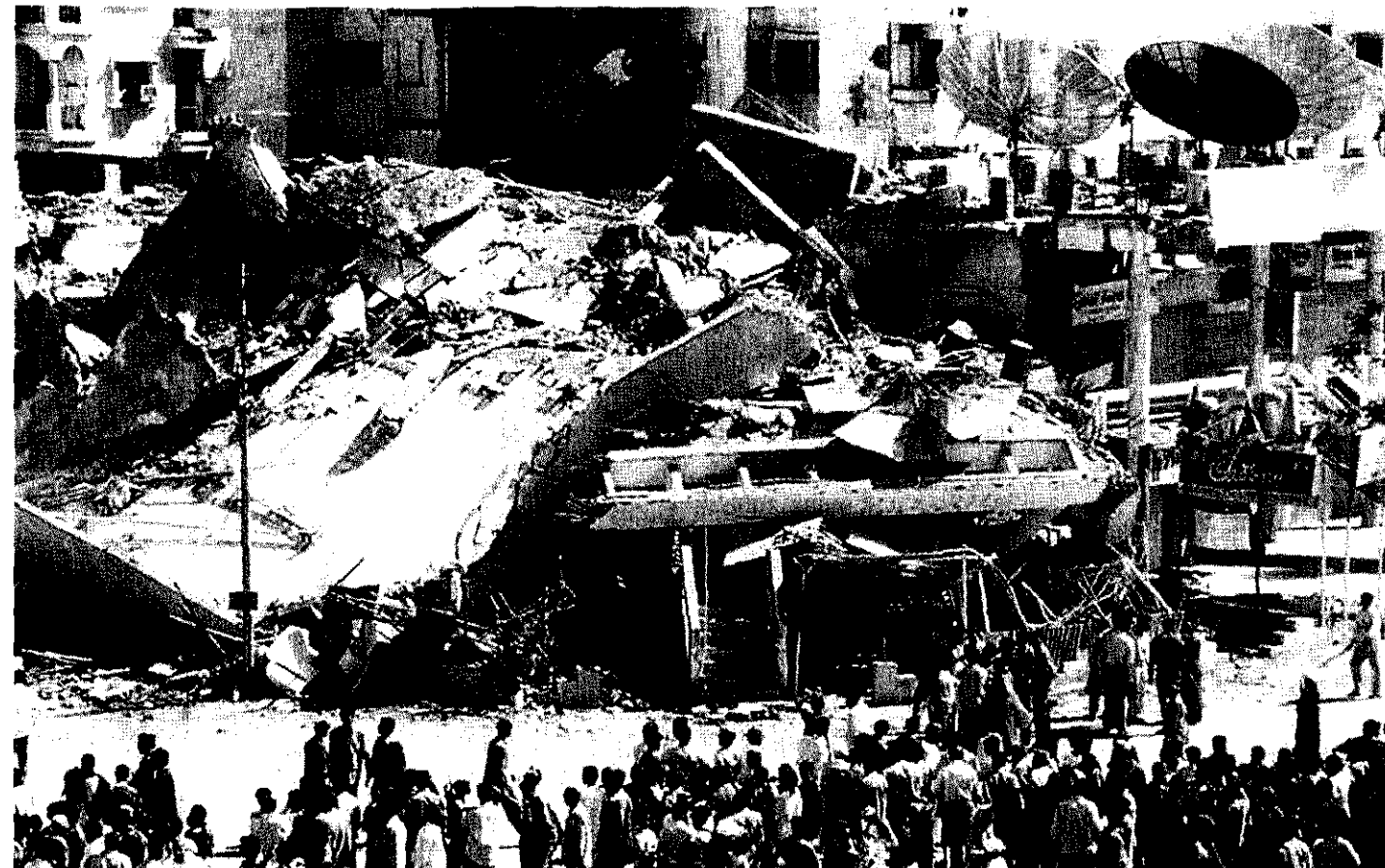
BLACK FRIDAY: People gather in front of a collapsed building in Ahmedabad in the aftermath of an earthquake on Friday. — Reuters
