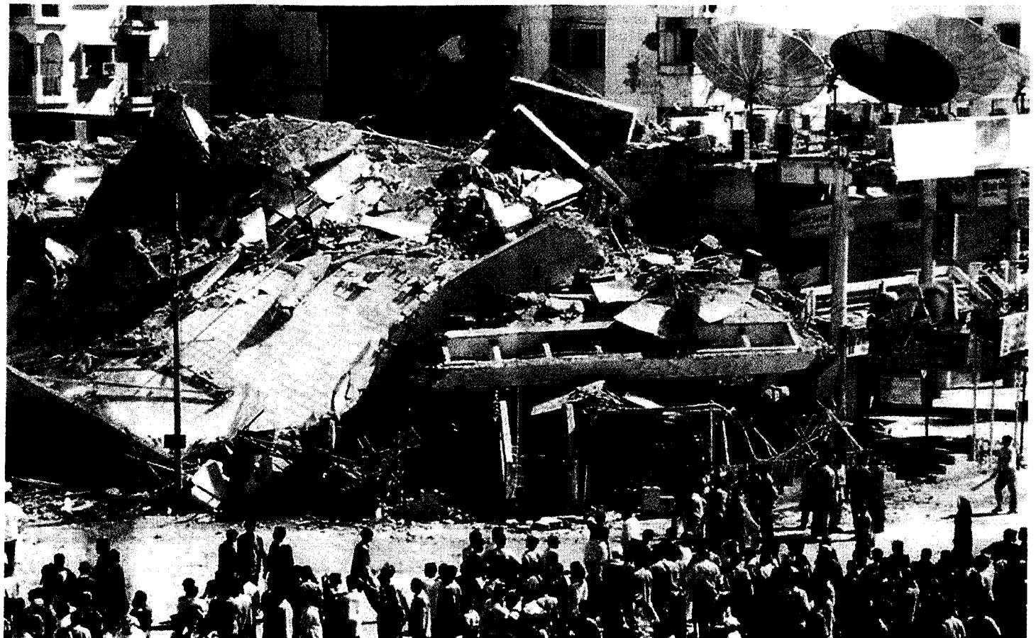
BLACK FRIDAY: People gather in front of a collapsed building in Ahmedabad in the aftermath of an earthquake on Friday. — Reuters
