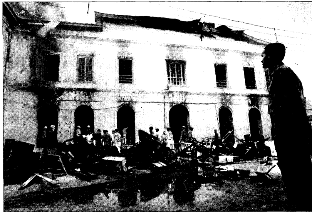
A securityman stands guard outside the damaged Assembly building in Srinagar on Tuesday.
