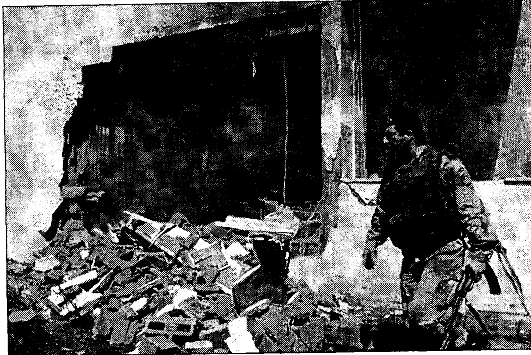
COUNTER ATTACK: A Palestinian policeman inspects the damage after an Israeli attack on a naval headquarters building on the coastal road leading to the Erez border crossing in the northern Gaza Strip on Tuesday. Israel launched missile strikes in the Gaza Strip on Tuesday. (Reuters)
