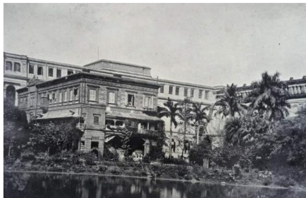
Figure 3.4 b) – The building Government School of Art, Calcutta with the structure of Indian Museum behind, as published in the Our Magazine . Collection – Govt. College of Art & Crafts, Calcutta. Courtesy – Soujit Das.
