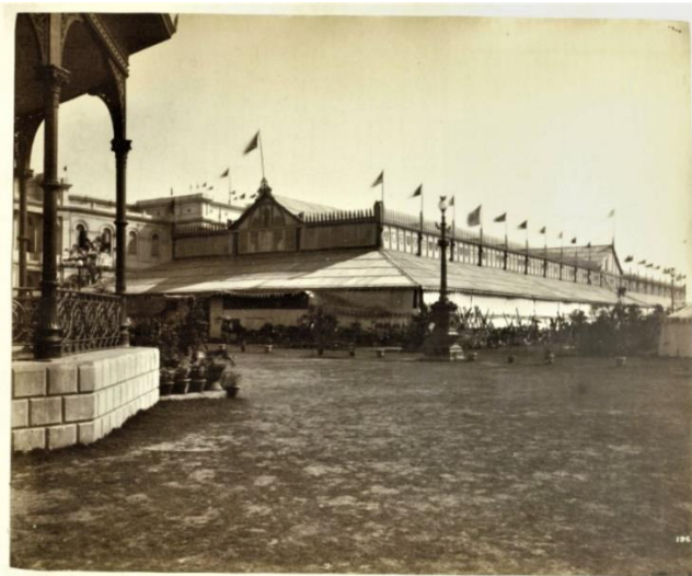
Figure 2.13 - View of the temporary exhibition sheds on Maidan for the Calcutta International Exhibition. 1883-84. Image Source: photographs taken by Mr. A. W. Turner, under the direction of the Government of Bengal. Printed and Published by the
