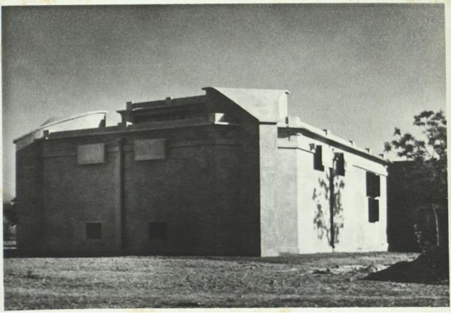
Figure 6.2 a) – Gradual evolution of the ‘Nandan’ structure, image from rear side of the building. Photographer Unknown. Image Collection and Source: RabindraBhavan Archives, Visva-Bharati
