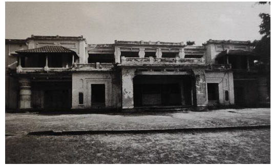
Figure 6.25 b) – Patha Bhavan (Old Library) building. . Image Collection and Source – Rabindra Bhavan Archive, Visva-Bharati
