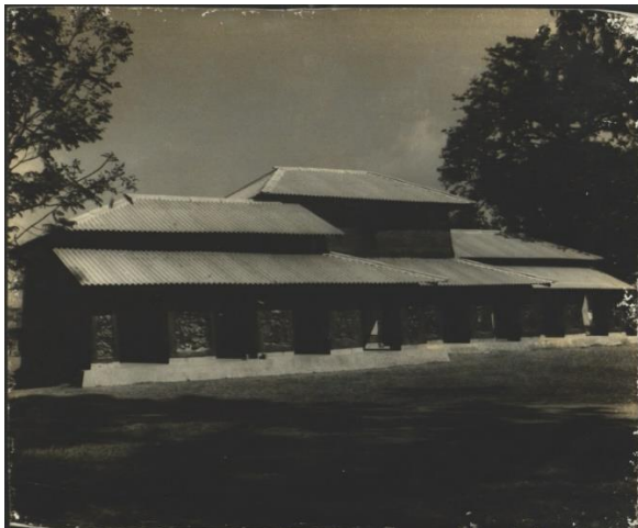
Figure 6.21 a) – Black House, Kala Bhavan. Photographer unknown. Image collection and Source – Rabindra Bhavan Archive, Visva-Bharati
