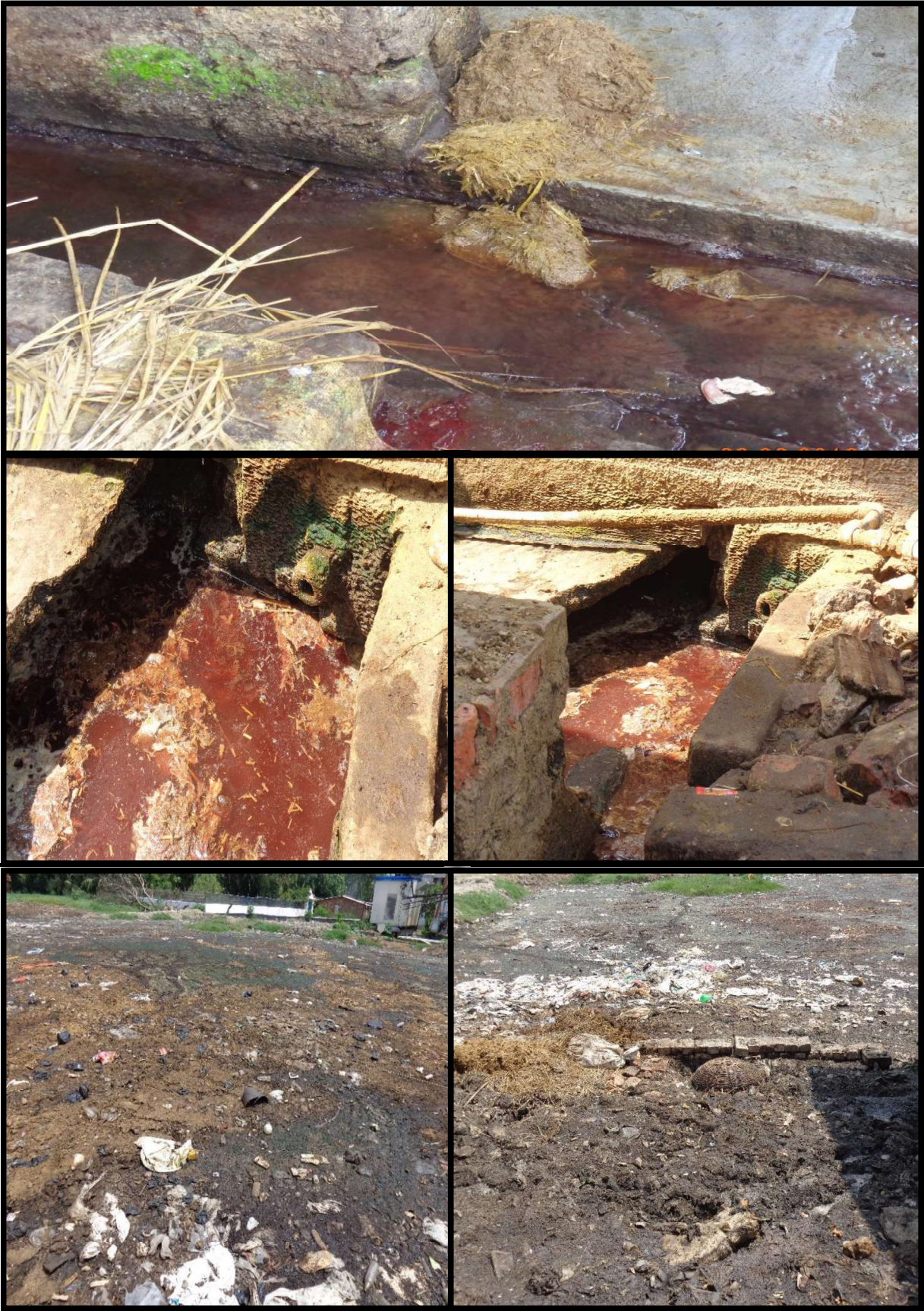
Figure 2: Choked on cattle blood channels and ruminal contents in open dumping sites.
