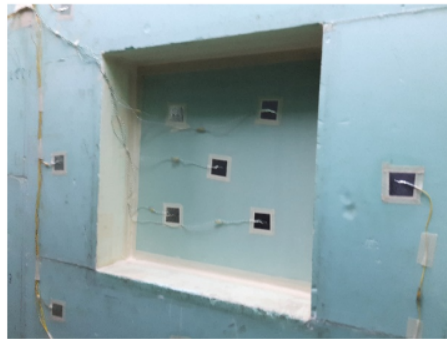
Fig. 2.29 50mm extruded polystyrene sample mounted inside surround panel of GHBC
