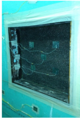
Waterproofing membrane applied surface facing metering box
