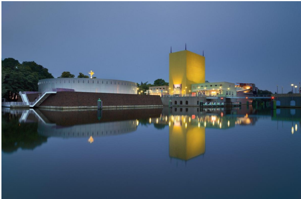
Figure 2.30 Groninger Museum astounding night building view
