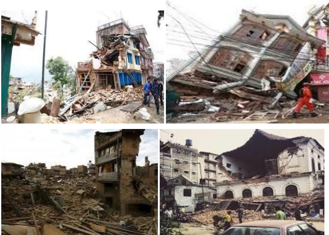
Figure 1.2: Severely damaged and collapsed buildings in Nepal earthquake
