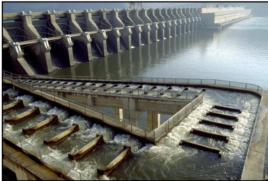
Fig 1.1.4, Typical Fish way or Fish Ladder
