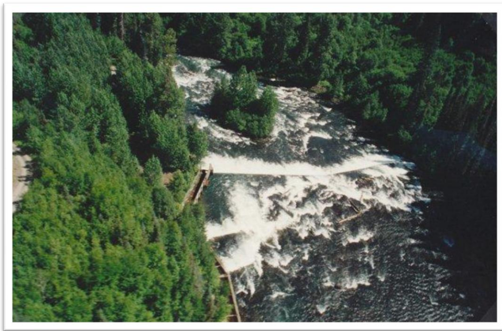
Fig.1.1.6, Aerial view of Meziadin Fish Ladders-1995
