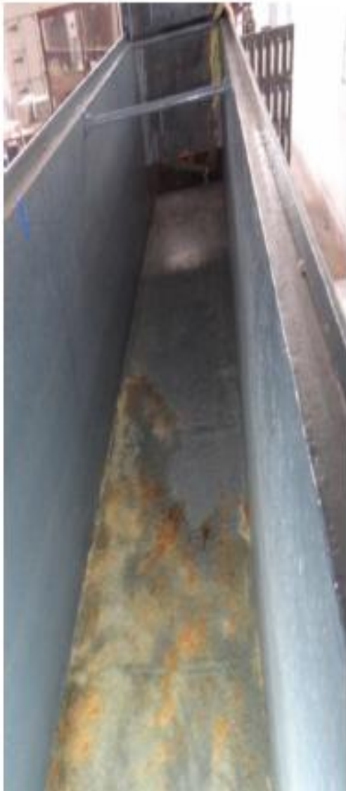
(a) Near the Inlet Sluice Gate
