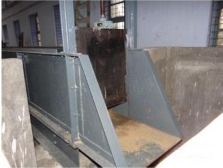
Fig. 3.1.4, end of Channel
