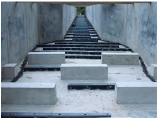
Fig 1.1.1, Concrete Baffled Culvert
