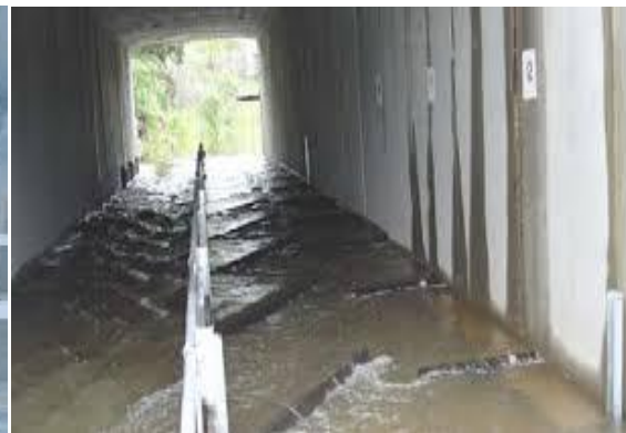
Fig1.1.2, Baffle Flume
