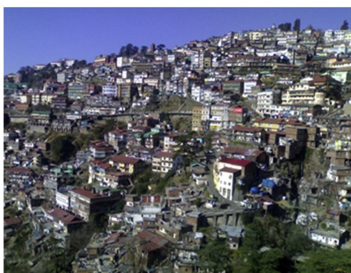
Buildings covering entire hill slope in Shimla town
