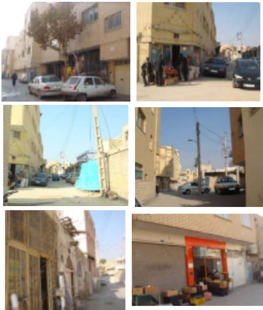
Fig 6.6 Condition of Khajoo neighbourhood
