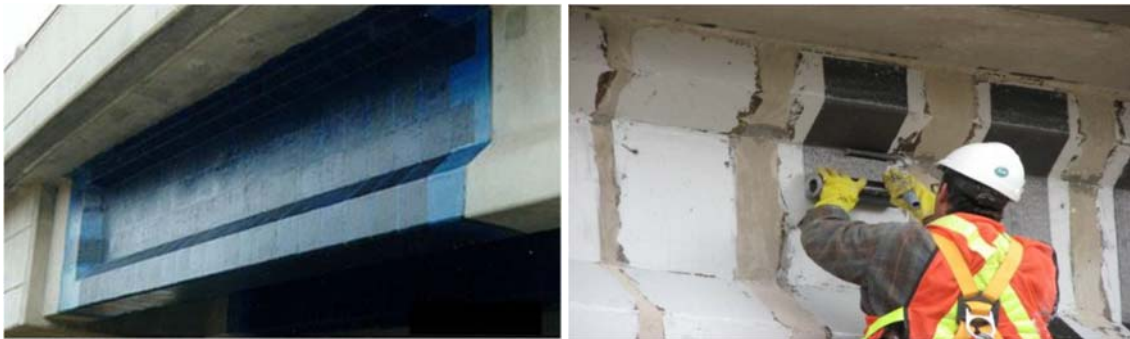
Figure 2.11: Shear strengthening of reinforced concrete using CFRP laminate
