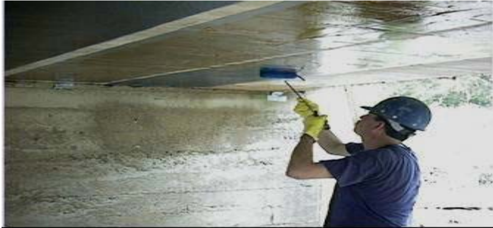
Figure 1.3: Fiber wrapping of the slab [15]
