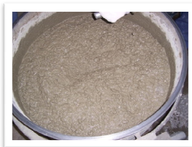
Fig 3.2.4 Preparation of PSC Mortar
