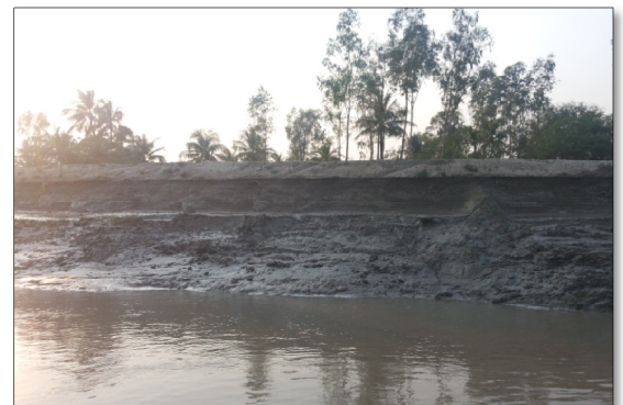
Figure- 4.4 : Sonakhali Site During Draw-Down
