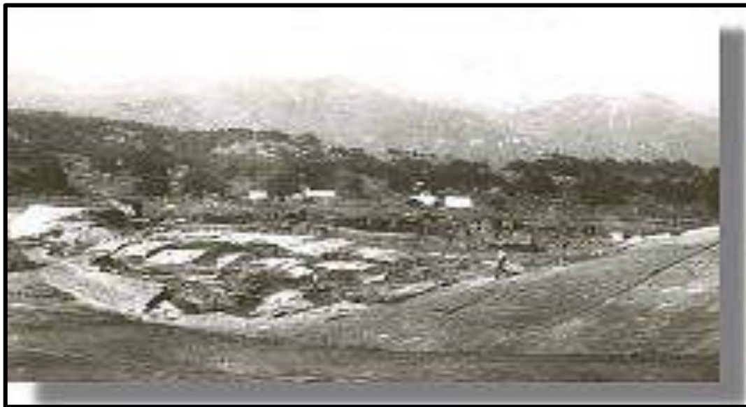
Fig 1.5 : Liquefaction failure of Sheffield Dam in the 1925 Santa Barbara Earthquake
