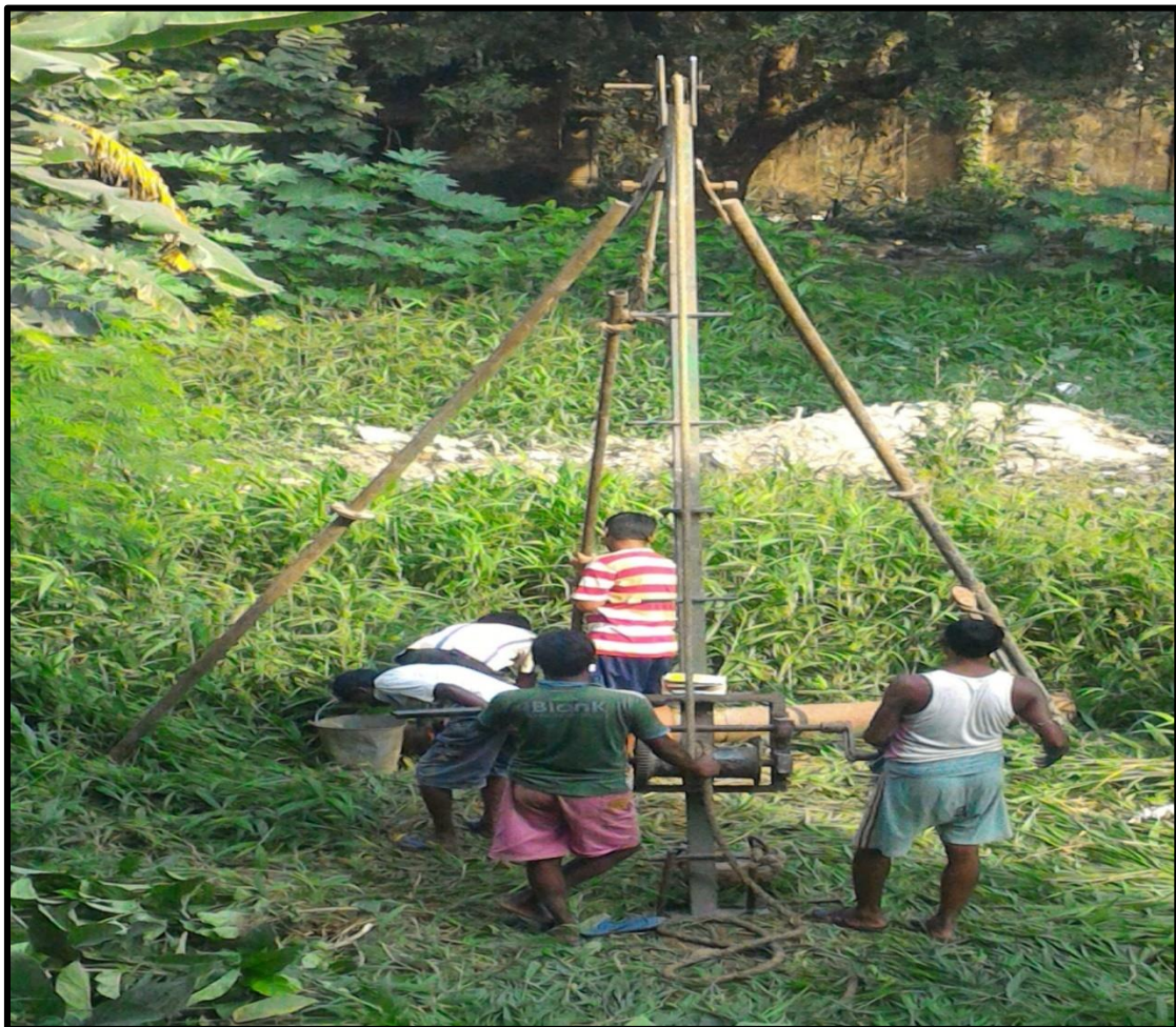
Fig 4.1 Boring work is going on for collection of sample
