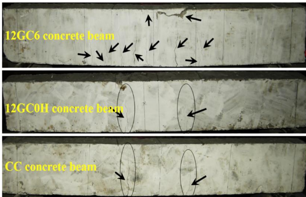
Figure – 5.18: Crack patterns of 12GC6, 12GC0H and CC concrete beams.
