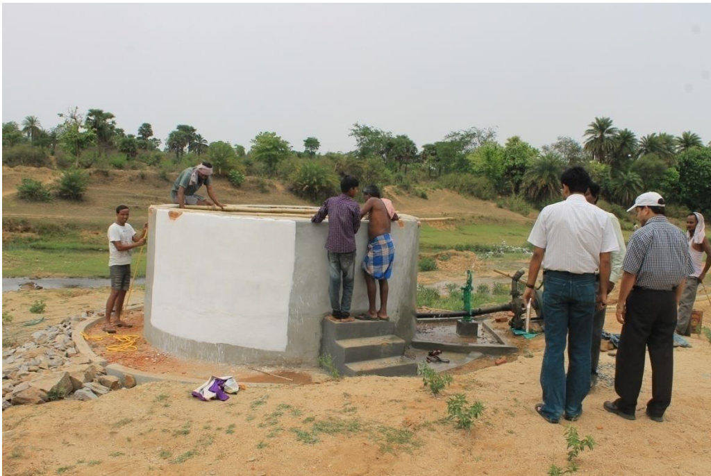
Photo 9.17: Constructed Collector Well
