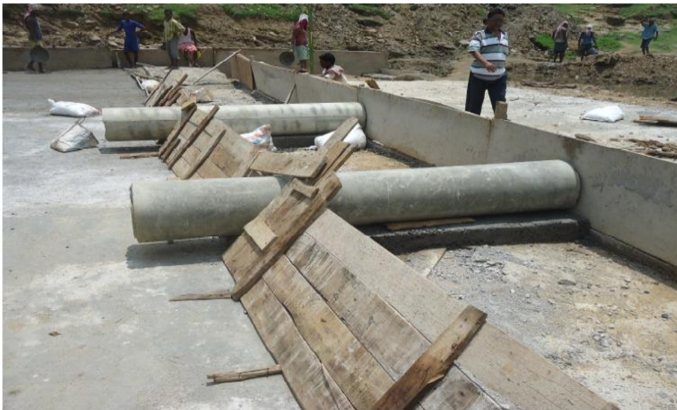
Photo 9.8: Installation hume pipe in check dam construction
