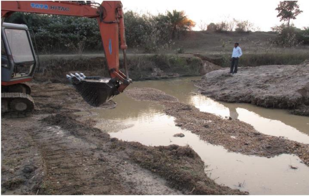
Photo 9.16 : Photo-Gravel packing in River Bed
