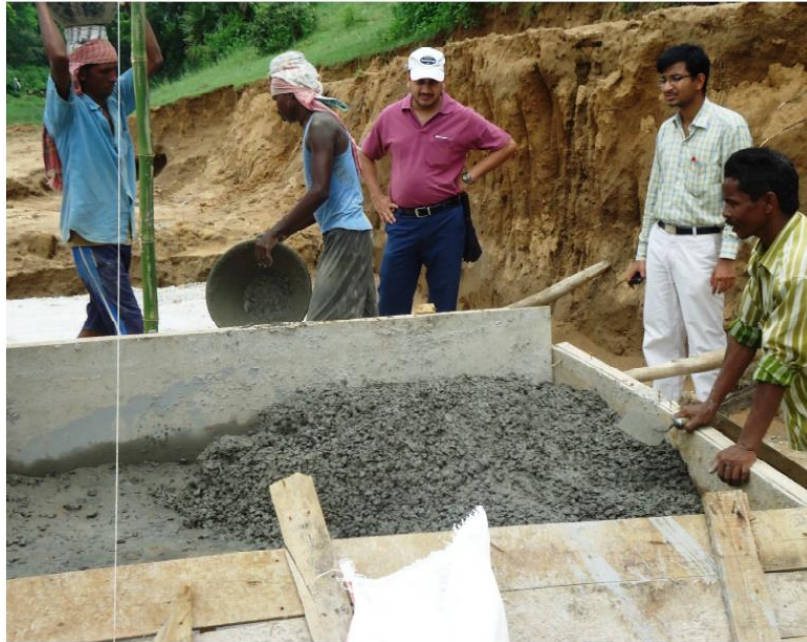
Photo 9.6 Construction of weir section of Dam site
