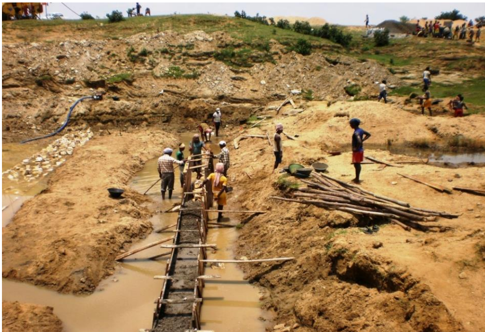
Photo 9.5 : Construction of Cutoff wall in upstream side
