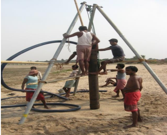
Photo 5.10 :Lowering of Casing pipe near Beldihi bridge
