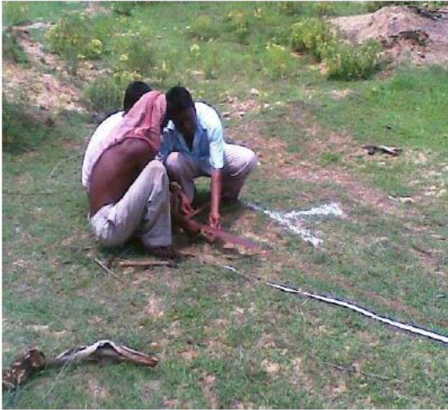
Photo 9.2 : Layout marking of construction site for check dam
