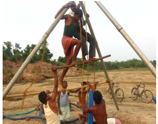
Photo 5.19 : Lowering Strainer pipe in Kudlung
