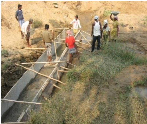
Photo 9.18 : Construction of Subsurface Dam
