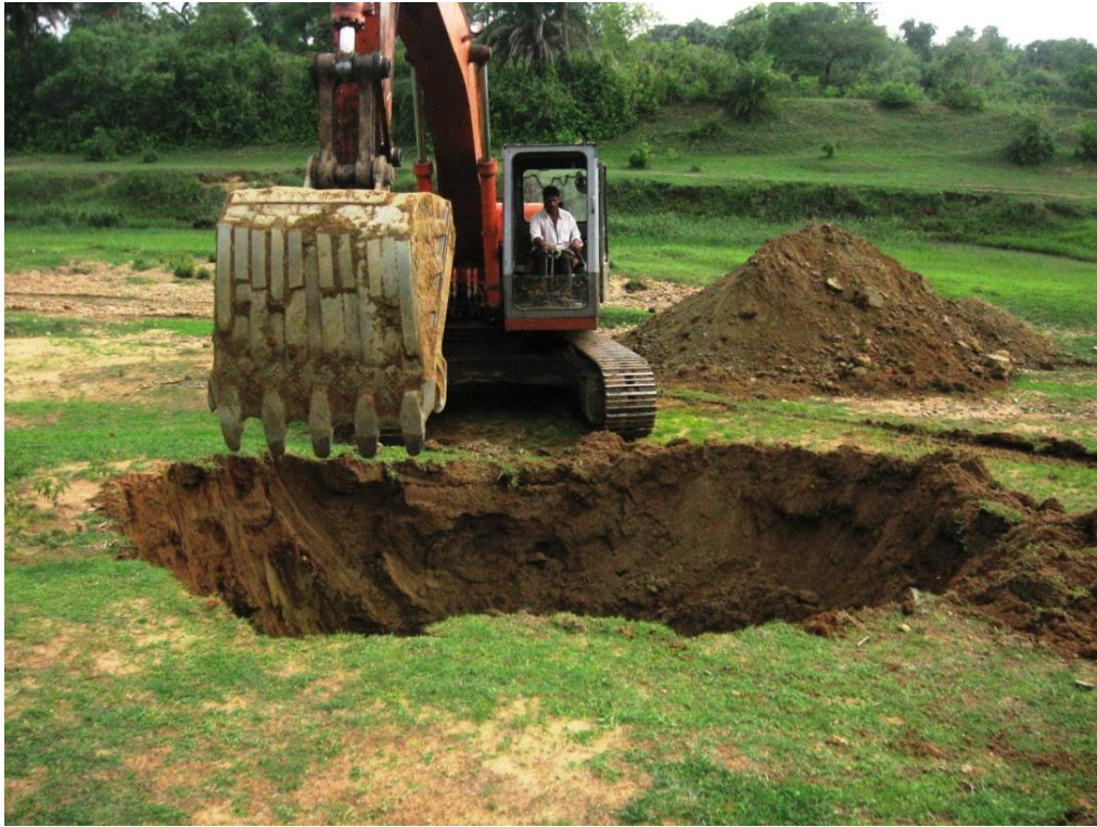
Photo 9.12 : Earthwork excavation for collector well
