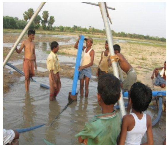
Photo 5.15 : Lowering of strainer pipe during at Joradihi
