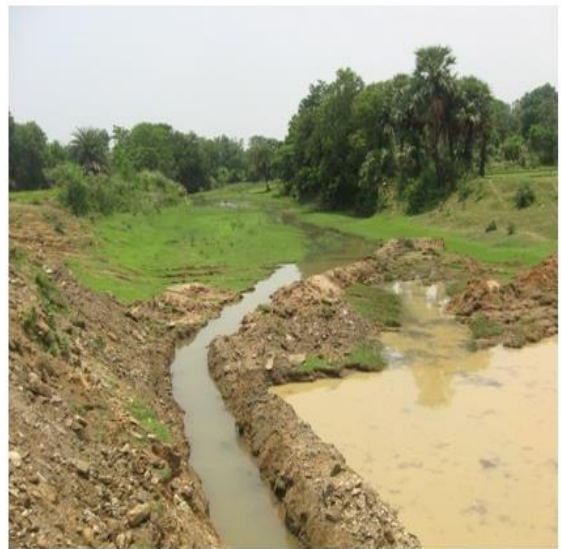
River condition before check dam construction
