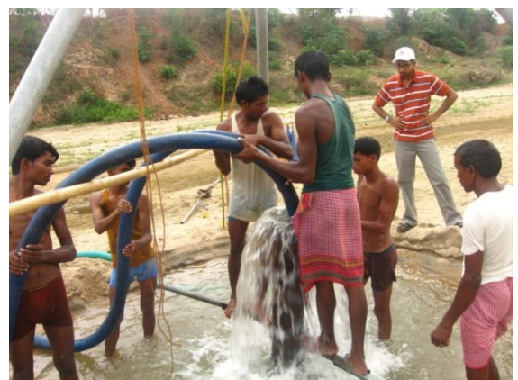
Photo 5.21 : Boring operation in kudlung
