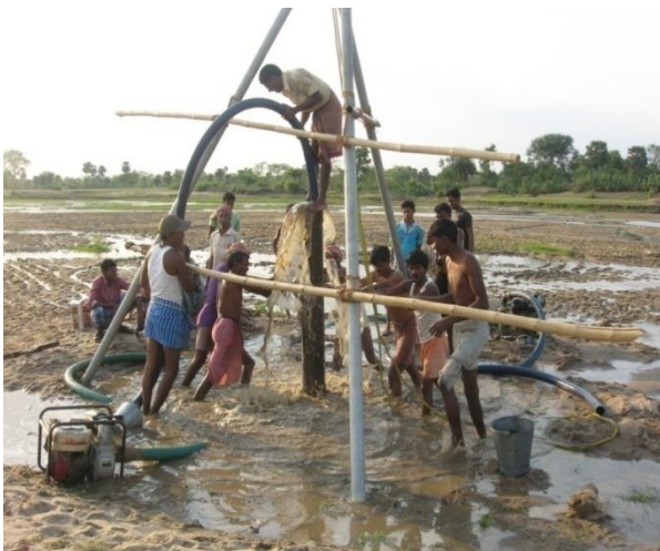
Photo 5.14 : Lowering of Casing pipe during Boring operation at Joradihi
