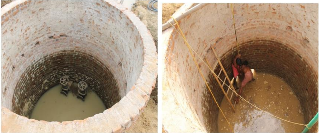
Photo 9.14 : Installation of Sluice valve
