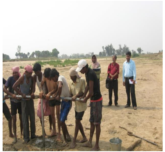
Photo 5.7 Slim Boring at Baligara
