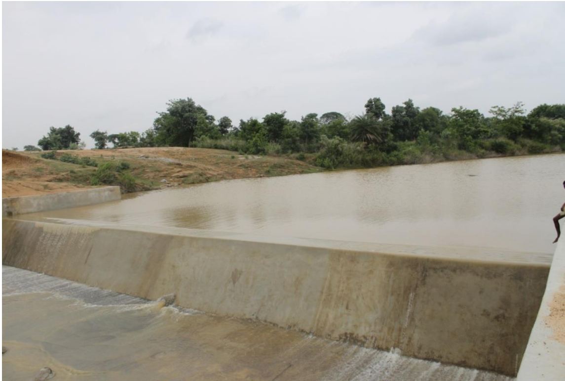
Photo 10.3: Increase in river water condition after construction of check dam in Monsoon, 2014
