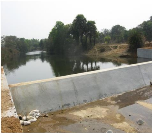
River condition after construction of check dam
