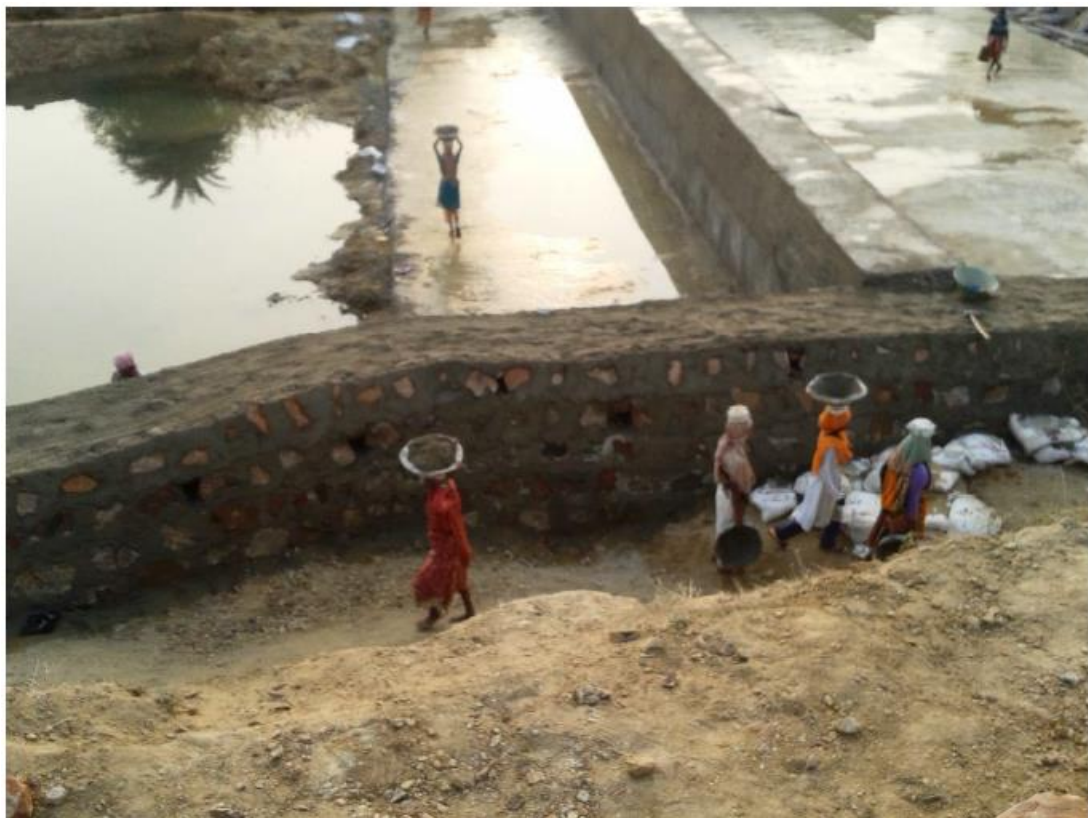
Photo 9.10 The construction of wing wall in Check Dam Unit
