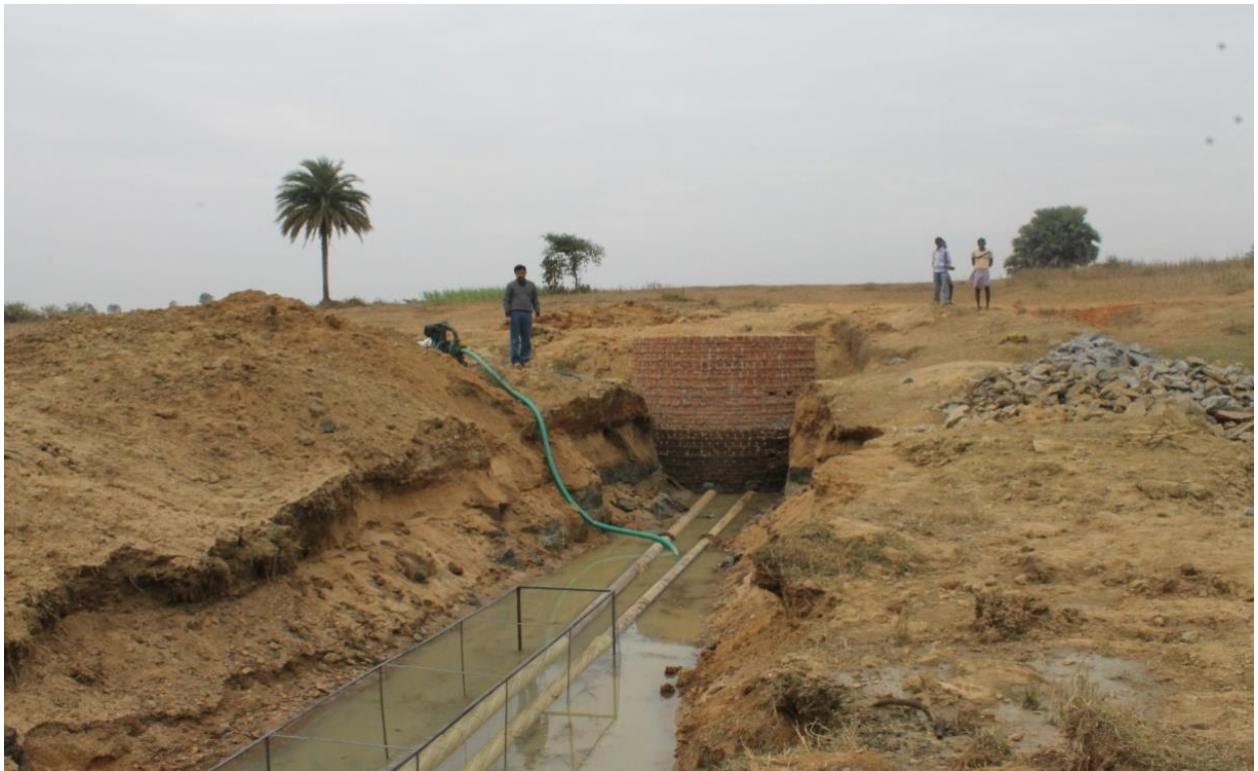
Photo 9.15 : Laying out of the strainer Pipe in the River
