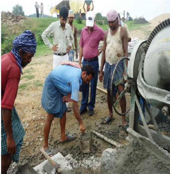
Photo 9.7 : Preparation of concrete test cube and its compressive strength for quality monitoring of the material section of Dam structure
