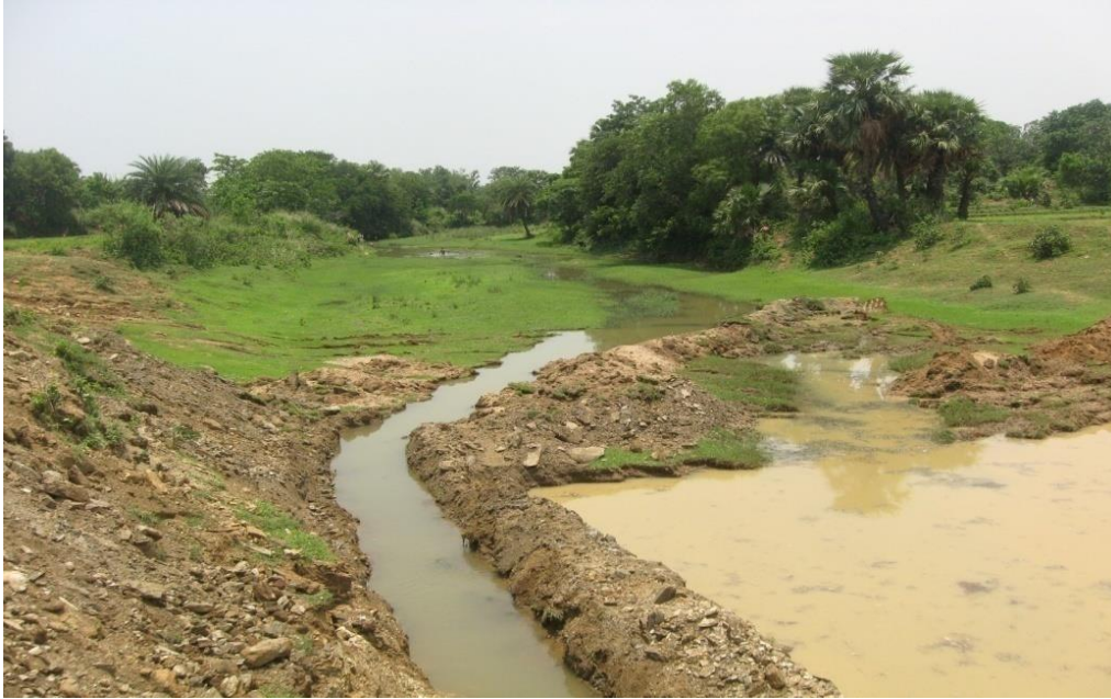
Photo 9.4 : Constructed Diversion channel
