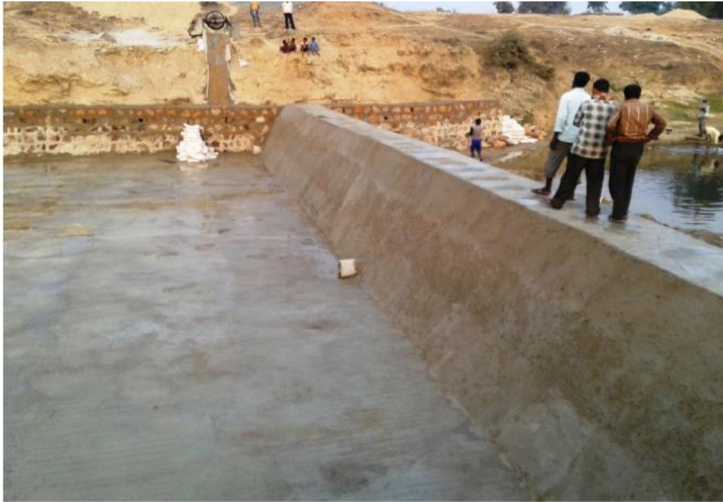
Photo 9.9 : The constructed weir section in Check Dam
