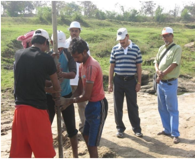
Photo 5.6 Slim Boring operation at Kotloi
