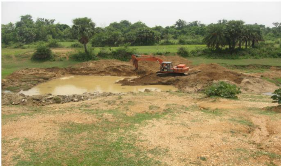
Photo 9.3: Earth work excavation for the foundation work of the check dam
