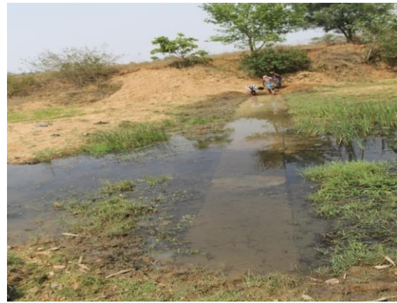
Photo 9.19 : Constructed Subsurface Dam and Its Effect
