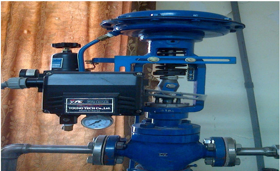
Figure 6.8: Pneumatic control valve with positioner in real time pressure loop.
