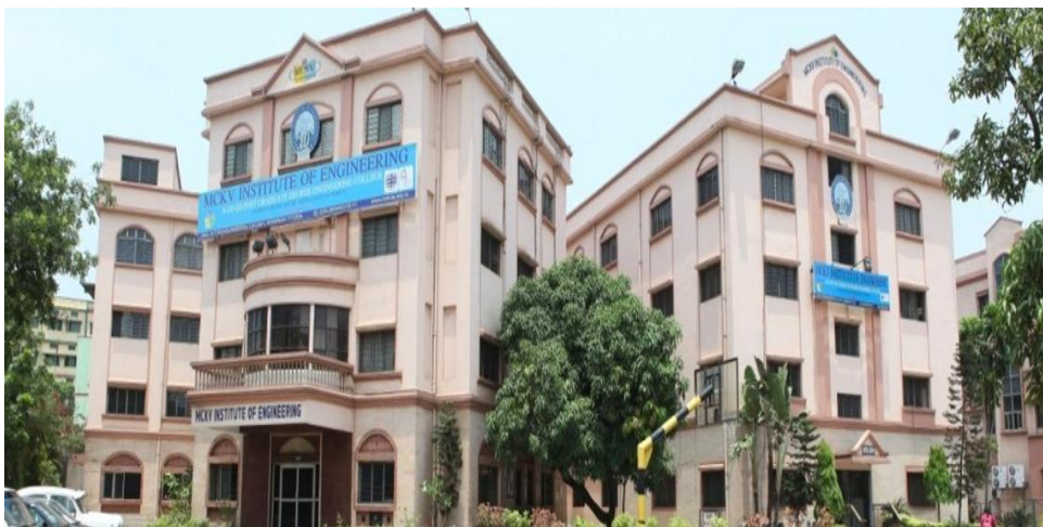
Fig. 5.39 : MCKV Institute of Engineering
