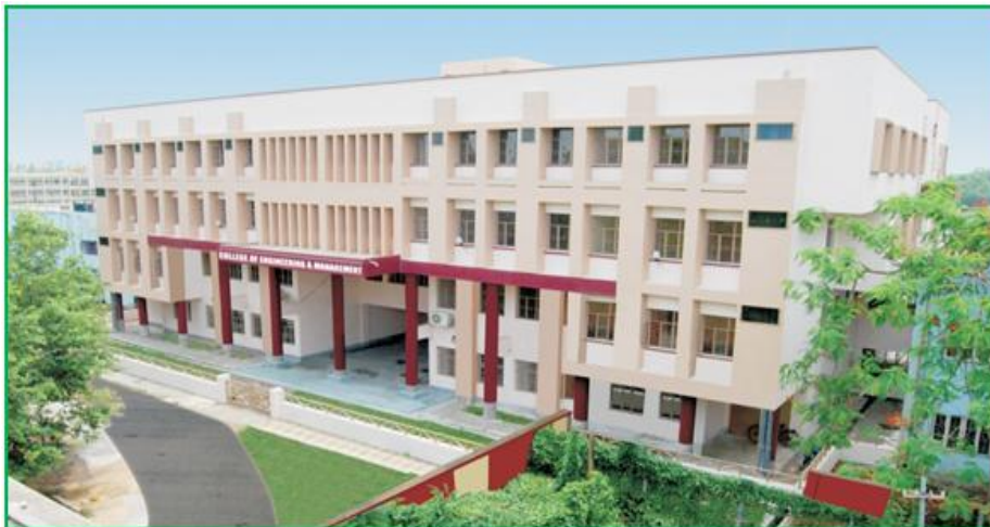
Fig.5.14 : College of Engineering & Management, Kolaghat
