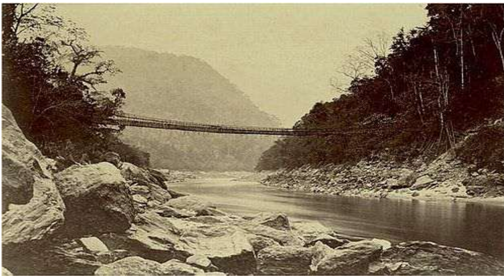
Samuel Bourne- Darjeeling Cane Bridge over Tista River
