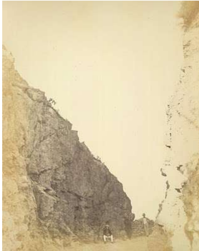
Darjeeling Hill Road Entrance to Pearson's cutting, 3 miles below Kurseong 1865 1
