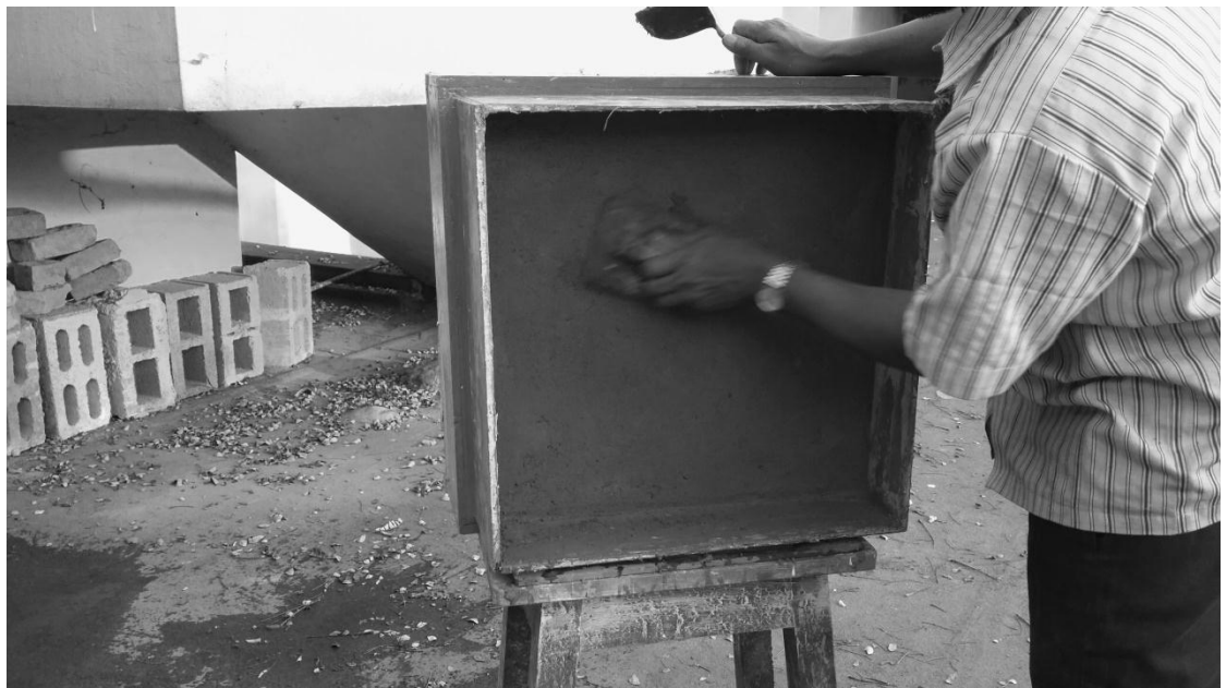
Fig.4.38. Construction of the brick wall sample under progress
