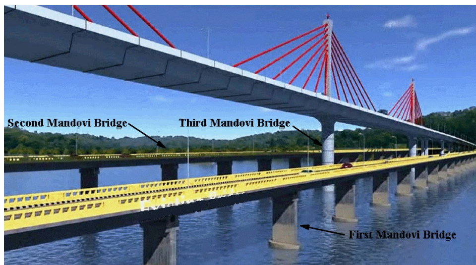
Fig. 1.2. Pier groups of First, Second and Third Mandovi Bridges in India.
