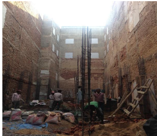
Plate 5.4: Construction activities contributing to the SPM Source: Field Survey
