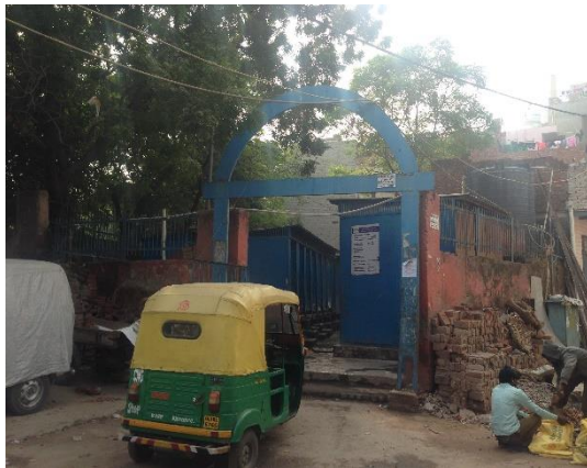
Plate 5.7: Community toilets in the Squatter Settlement Source: Field Survey
