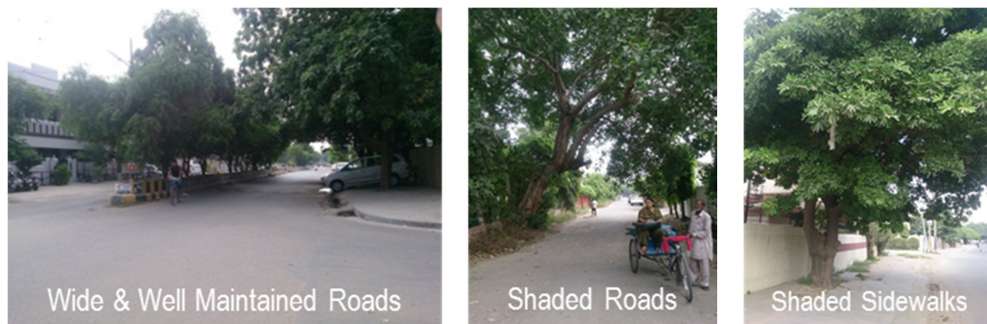
Plate 4.7: Condition of Roads and Sidewalks, Ranjit Avenue, Amritsar
