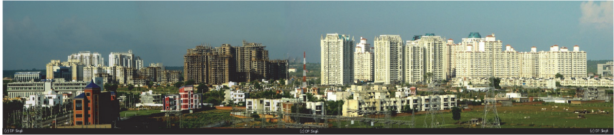
Plate 3.1: View of residential projects along NH-8, Gurugram
