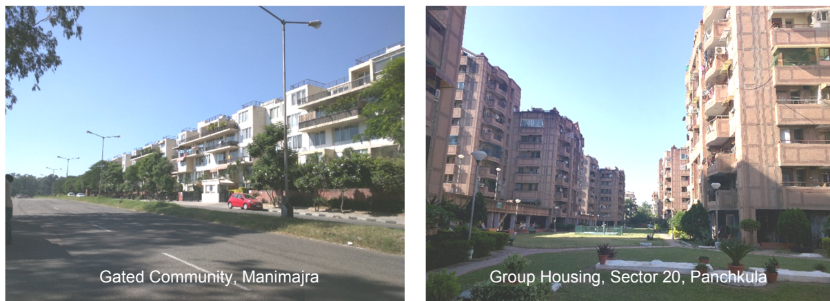
Plate 4.11: Medium Rise Structures, New Areas, Chandigarh Urban Complex
