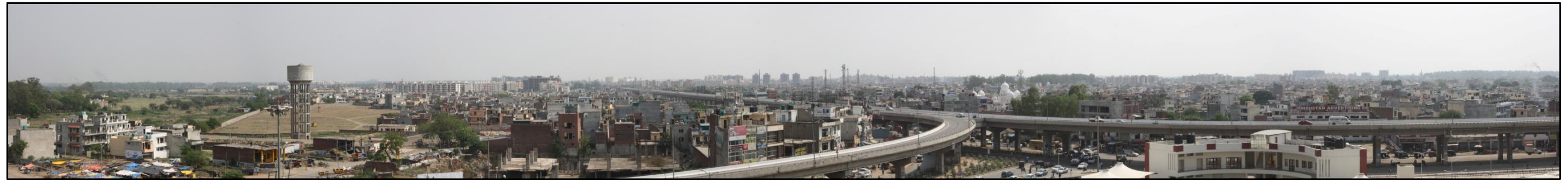
Figure 4.33: Zirakpur - the dense ribbon development along the main highway / Zirakpur fly-over
