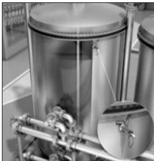
Figure 7.3: Schematic Arrangement of Point Level Sensor
