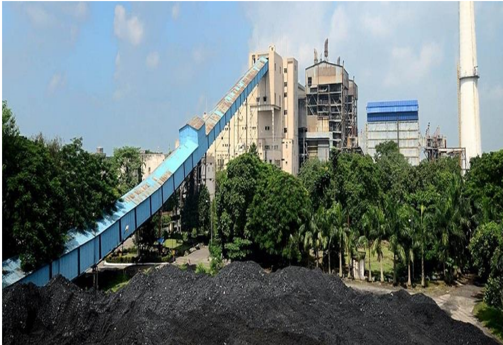
Figure 6.3- Power plant ( Source - Titagarh thermal power station )
