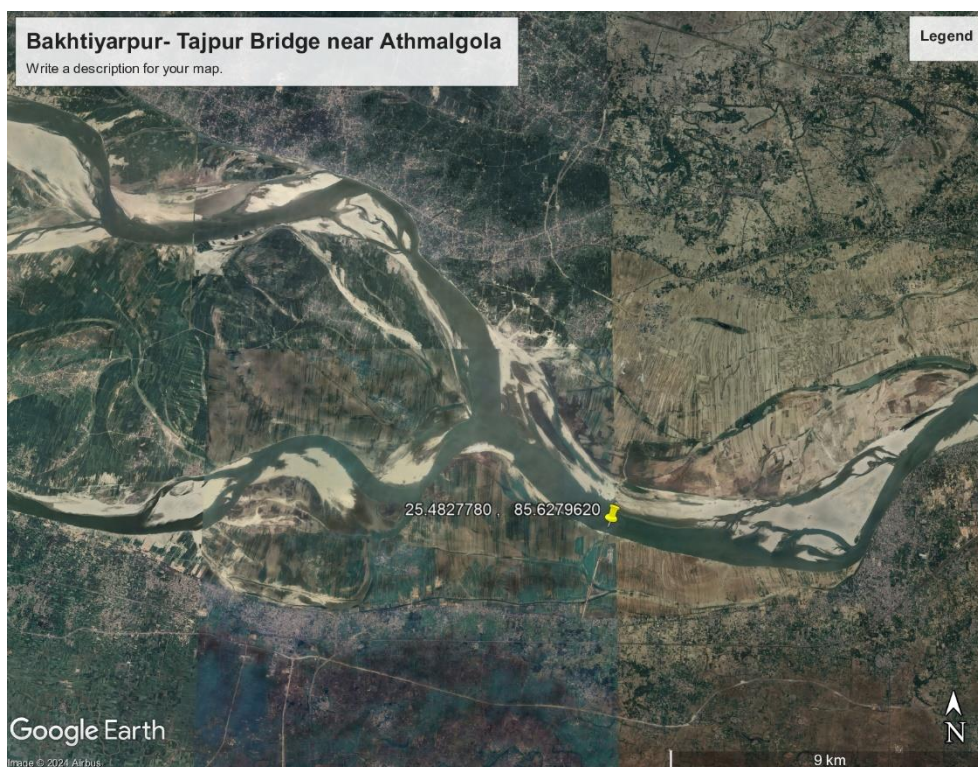
Fig.4.4.10. Bakhtiyarpur- Tajpur Bridge near Athmalgola
