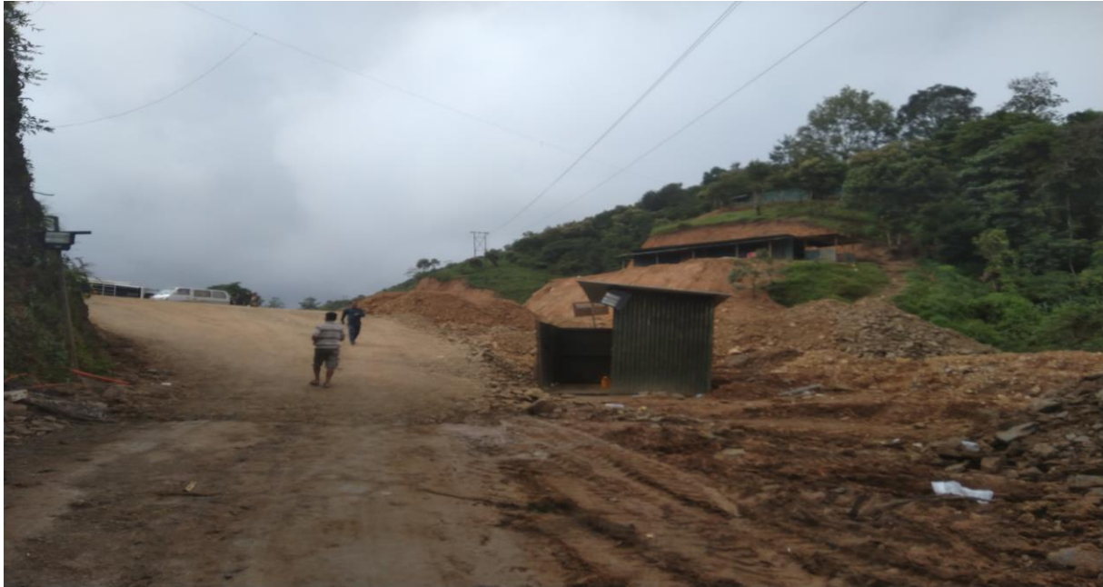
National Highway 39: Widening of Imphal to Moreh Stretch (2019)
