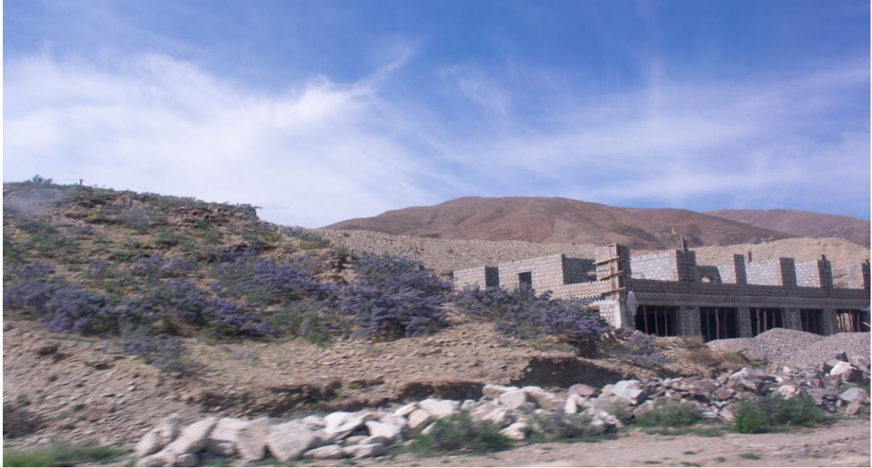
New houses being constructed along the old Southern Silk Route in Tibetan Autonomous Region (China), 2019.
