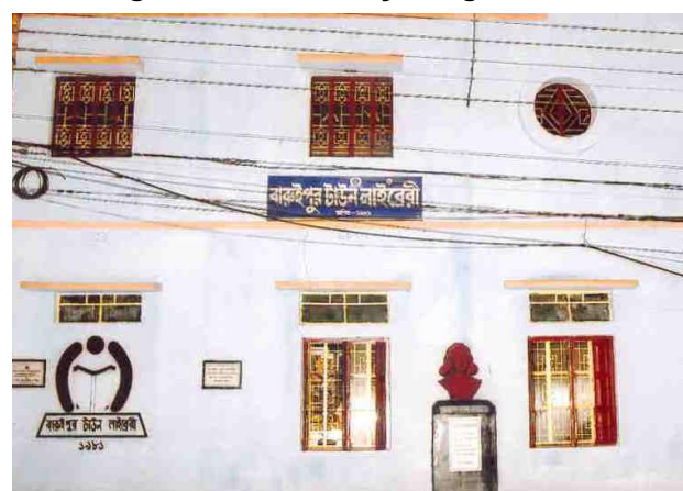
Baruipur Town Library, Baruipur
